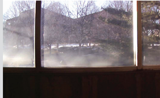
Silicate runoff from concrete facades.
