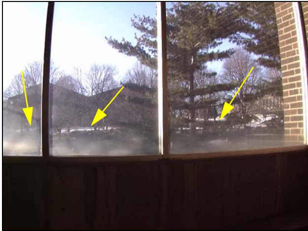
Figure 9: Visible gray haze due to deposits on glass from concrete runoff. Implementation of conventional cleaning procedures failed to remove deposits.
