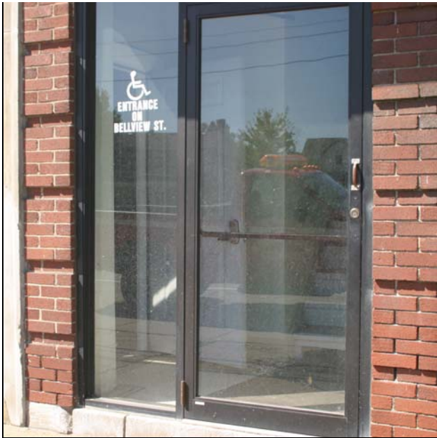
Figure 1: Entrance door on a municipal building located within 30 feet of a busy roadway.
