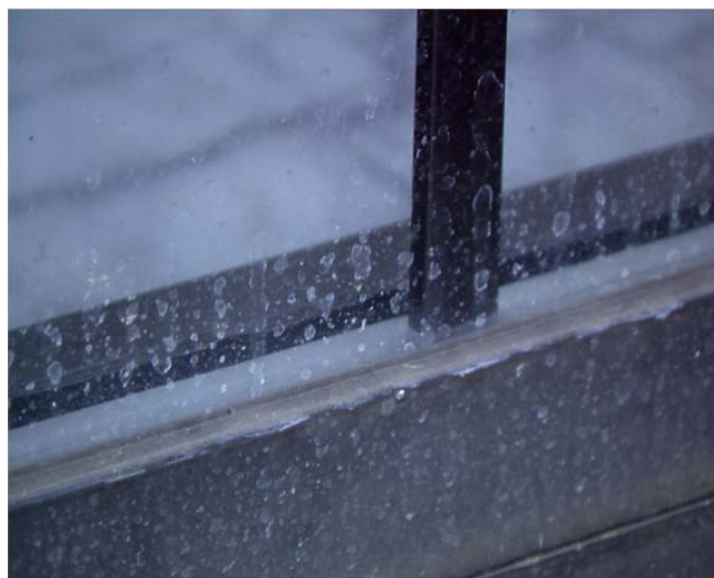
Figure 15 Hard water spots containing silicate materials after normal attempts at cleaning.
