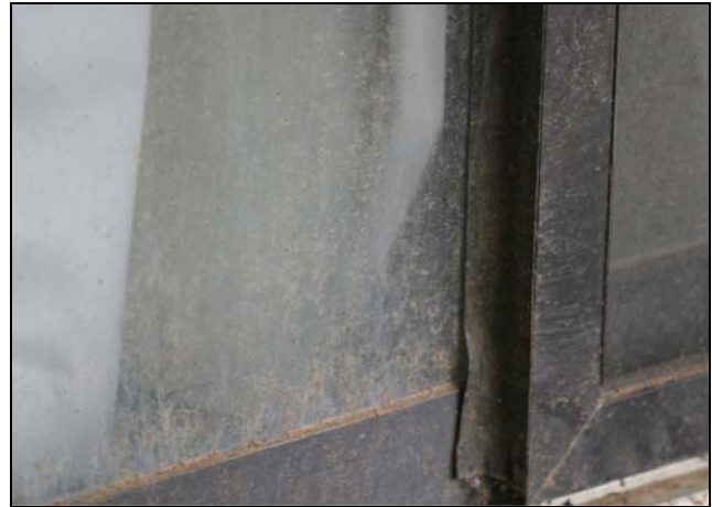
Fig. 5: Close-up view of dirt and soil on window at Virginia vacation home.
