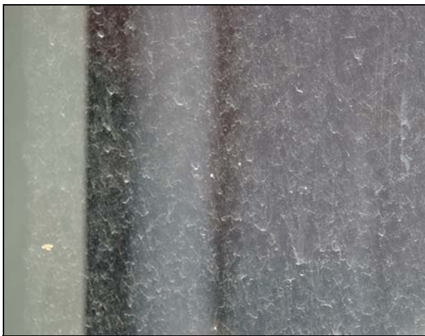
Figure 2: Close-up view of municipal building entry door reveals a significant accumulation of dirt and soil.
